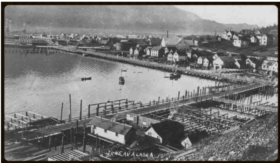
Willoughby Avenue under construction, looking north from Telephone Hill, 1914.
