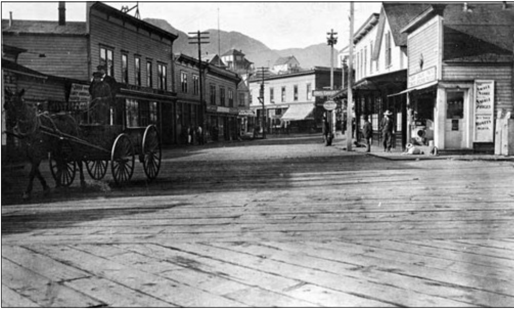
Front Street, looking west from Franklin, about 1910. Wooden planks on gravel fill. ASL P01-2240
