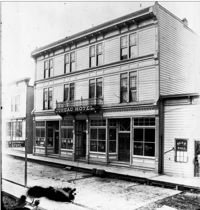
Second Street between Seward and Franklin. About 1908. Wooden planks on soil sub-grade. ASL P87-0952
