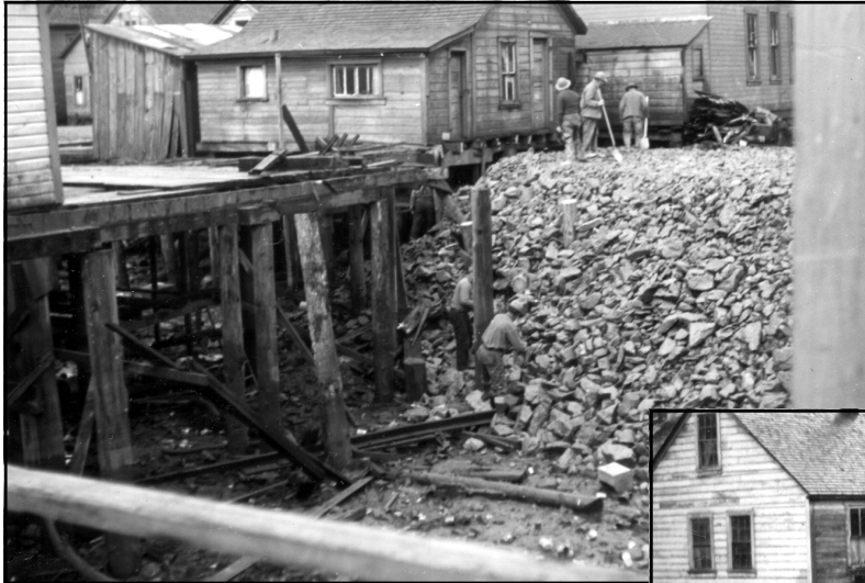
Civilian Conservation Corps workers working on the fill in the Village, 1941. (JDCM 2004.58.0009D)
