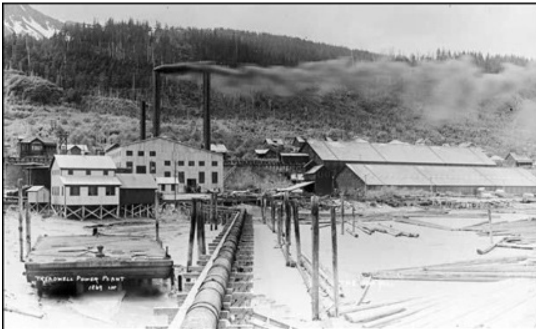
Treadwell, about 1915, from near the saltwater pump house. The central power plant is on the left, and the 300 mill on the right. The timber-trestle-supported pipeline in the center conveyed water from the pumps to shore for mills and fire-fighting. ASL-P75-422
