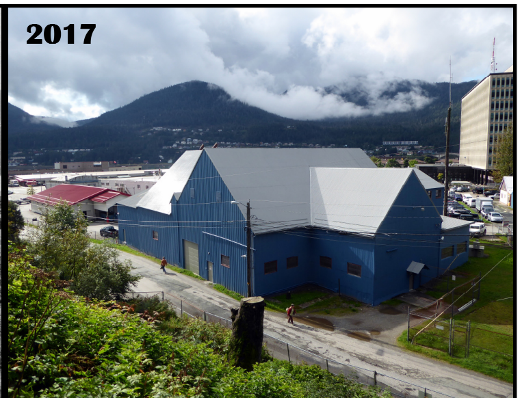
The Gold Creek plant, looking down to Capital Avenue from the "Fosbee" stairs. From 1914, the original plant (see left) was modified and expanded in stages to its current installed diesel/hydro capacity of 75,000 kW. The hydro turbines operate only in the Spring to Fall interval, when Gold Creek's flow is sufficient. AEL&P
