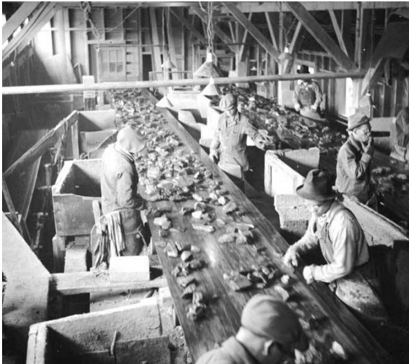
"The rock from the crusher runs over belts where workmen pick off the quartz and put it on a conveyor allowing the waste rock to keep on moving." ASL-P306-027
